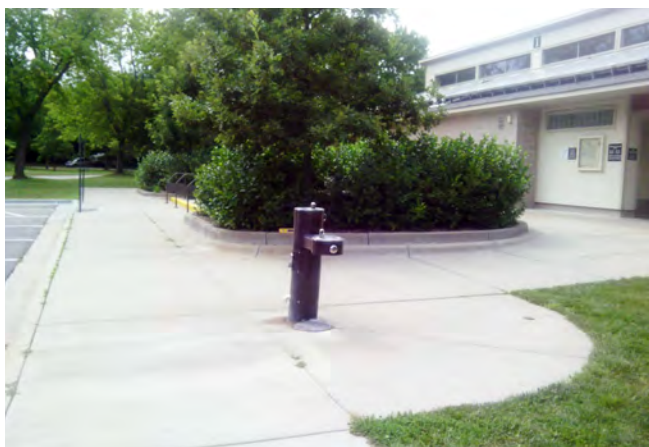
Accessible drinking fountain at shower building number 1
