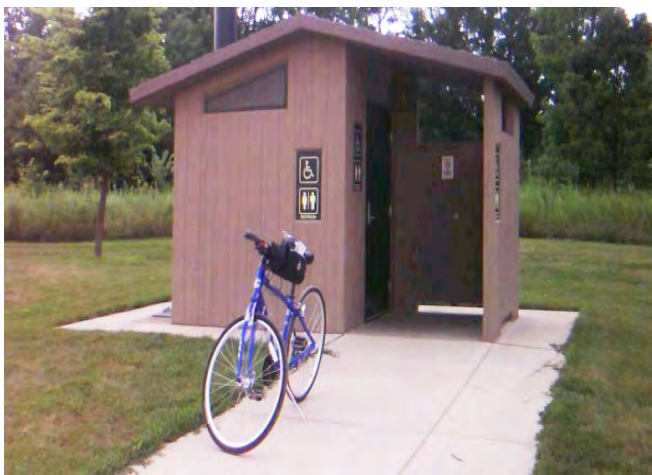
Accessible restroom at the dog off-leash area
