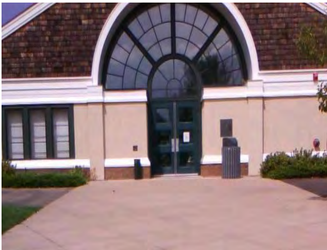
Accessible route to entry from parking
