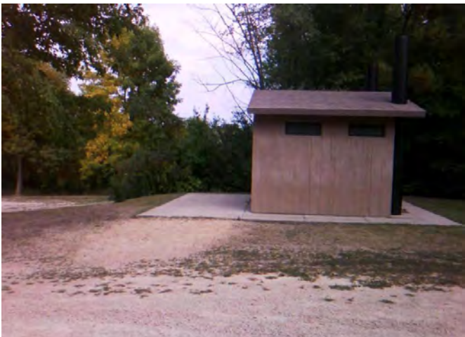
Access route to restroom at park entry
