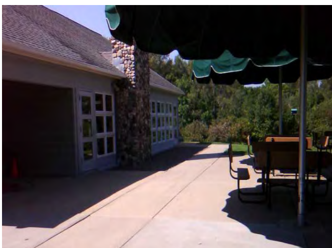
Accessible route at back patio of Visitor Center
