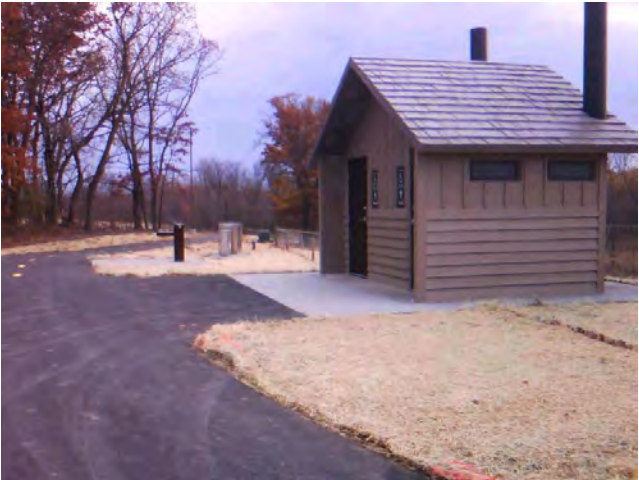
Access route to restrooms from parking lot
