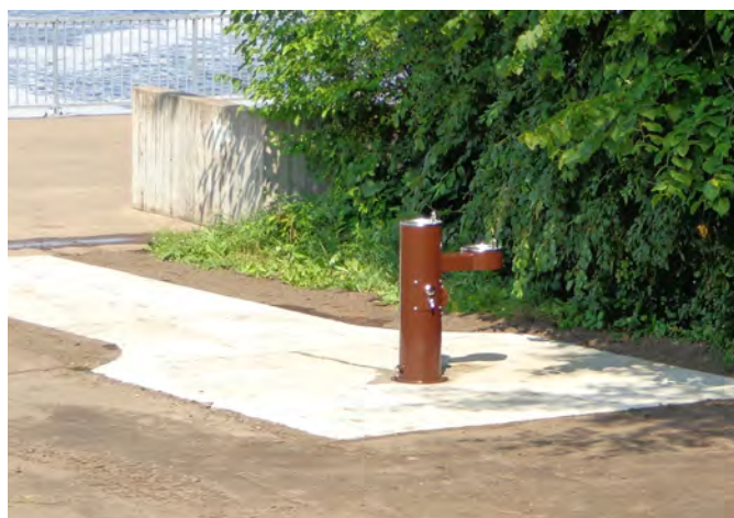
Accessible drinking fountain
