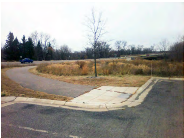
Pedestrian ramp at dog off-leash area
